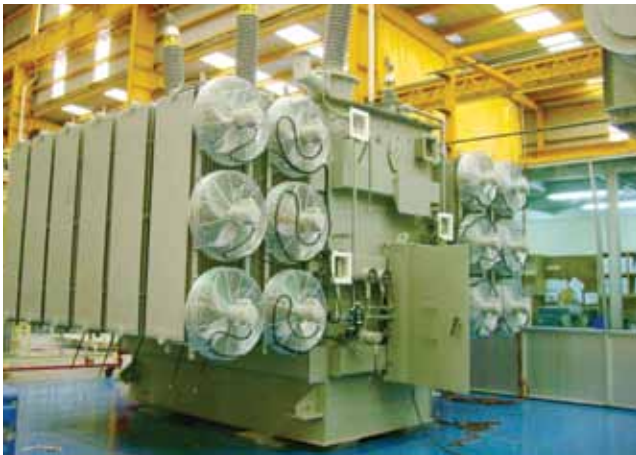
JOHN DEERE MOUNTAIN HOME SUBSTATION Glenns Ferry, ID 28/37.3/46.6 MVA – 138kV
