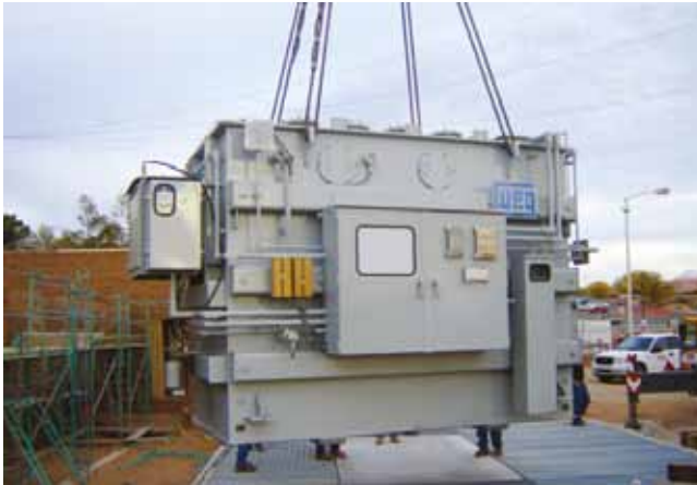
UNIVERSITY OF NEW MEXICO Albuquerque, NM 24/32/40/44.8 MVA – 115kV
